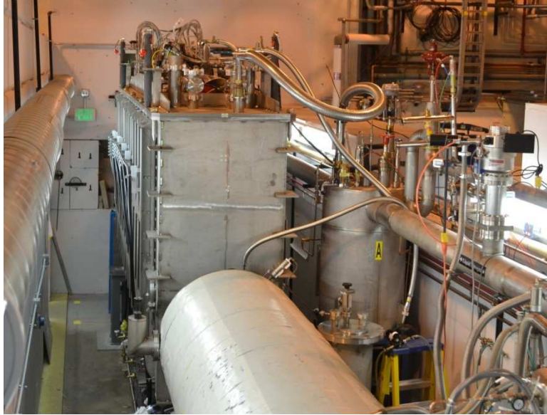
Figure 2: The reconfigured ATLAS Booster area with the new cryomodule (rectangular structure) coupled to a cryomodule of the previous generation (white, circular structure).
